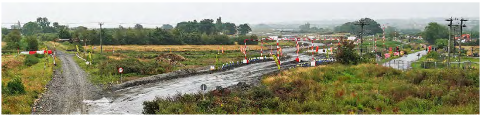
above looking southeast from Doddershall road bridge with the former lifted GCML leading to BRC on the left and showing the vast area covered by HS2 construction works to the south of BRC (right of photo) and the reason Station Road is closed
