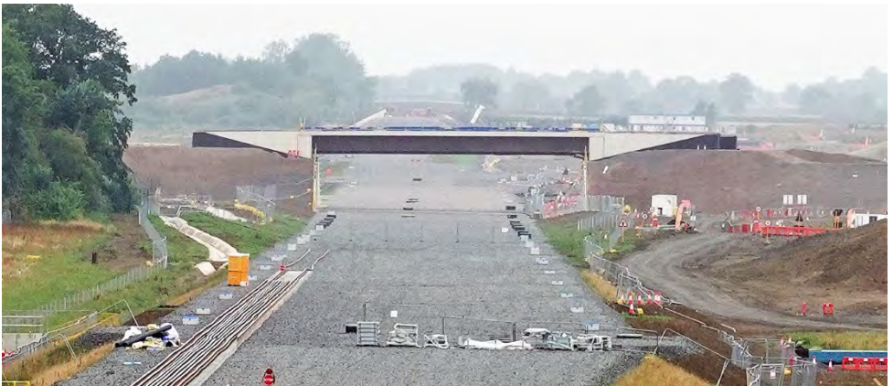
below a closer view looking west of the Steeple Grange to Calvert road overbridge and ramp up to cross HS2 and the road overbridge to be demolished middle distance, also showing the wide trackbed
