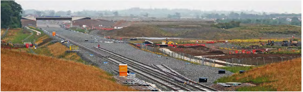
above looking west from Queen Catherine road showing the widened EWR trackbed and sidings being laid to the maintenance facilities
