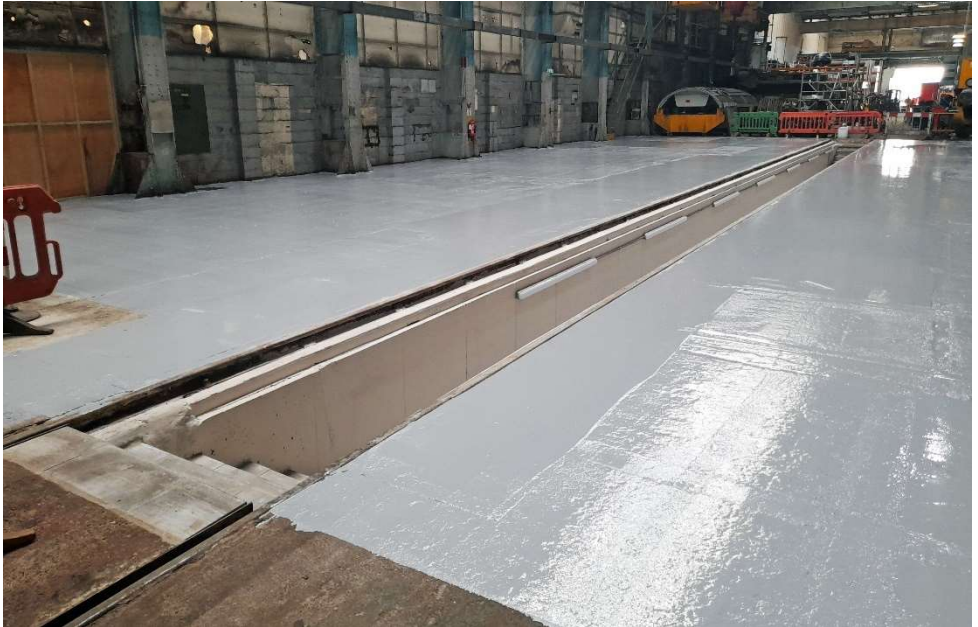
above Bay 3 Inspection Pit 15.01.25 (Carl Watson)
