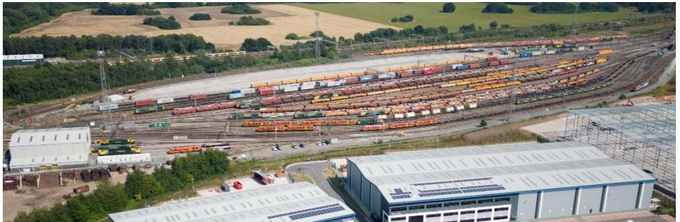
above An aerial view of Crewe Basford Hall from a couple of years ago (15.43) 16.07.22 (Darren Bailey)
