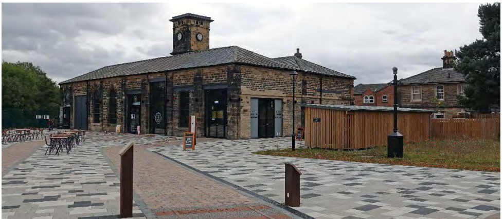
above the Goods Shed & clock tower from the paved former yard
