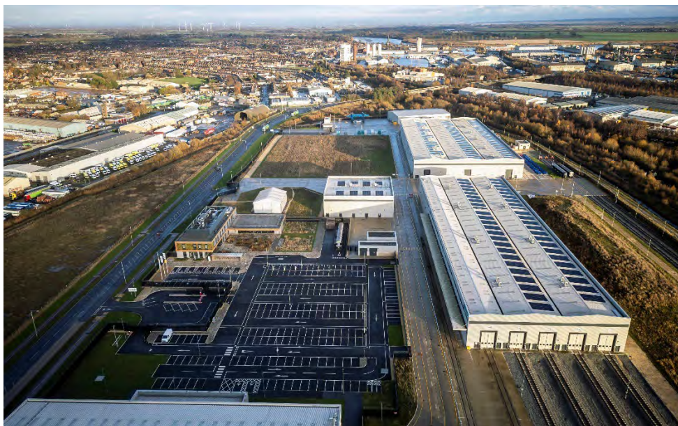
looking east with the A161 Tom Pudding Road on the left and centre top the 'salt & pepper pot' water towers and football ground either side of the mainline, beyond which is the station
