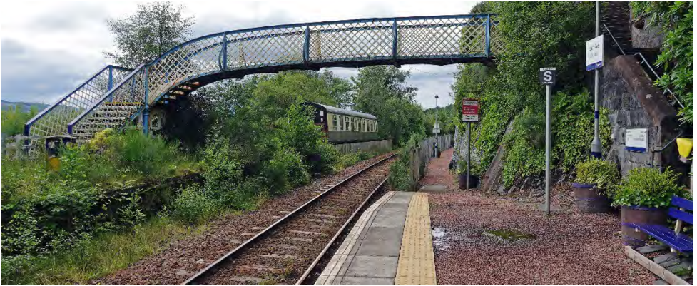
above looking southwest from the station with the overgrown original platform to the left to which the footbridge gave access
