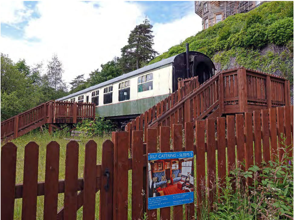
The coach was initially used as a café then sold to become self-catering holiday accommodation from 2009 but is now out of use and the area around the coach is becoming overgrown. This is a great location with rail access and considering where some coaches have recently been converted for glamping, it seems crazy to allow this coach to deteriorate. It would even make a great quirky annex to the hotel.
