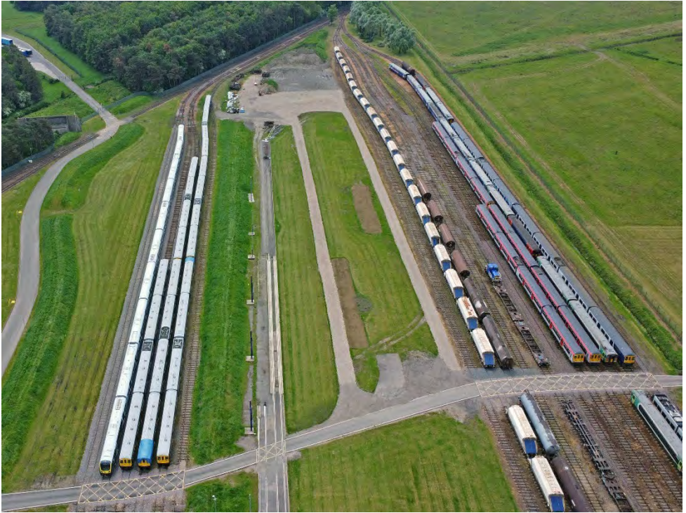
above eastern side looking south left to right and bottom to top 701004, 769913, 769946 + 769932, 739947 + 769928 + 769922 then on right south of the cross roadway, 21 JGA hoppers 19199/71/97/85/96/70/83/95/76/86/73/72/94/93/74/92/80/78/84/88/90, KBA barriers 85933 + 85936 + 4 JIA hoppers, IKA 33.68.4909.552-4 + 01544, 769452, 769007 + 769003, 153365/56/81/75/16/59/60/24/30/32/58, 319371 + 319454 (gap) 153363/71/83 (gap) TDA 86932 note the roadway leading to the former compound is on the left crossing the circular test track (12.59) (Gareth Taylor)
