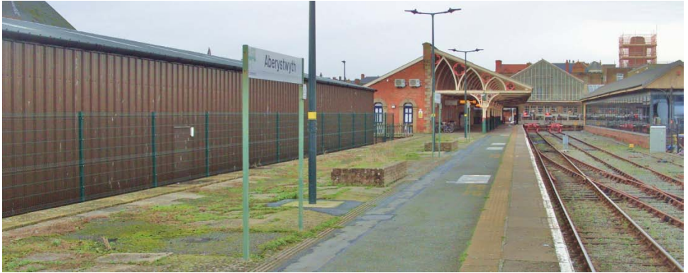
above & below looking west along the NR platform of Aberystwyth station with the new shed occupying the former VoR terminus, for comparison see photos on p25 July 2019 issue
