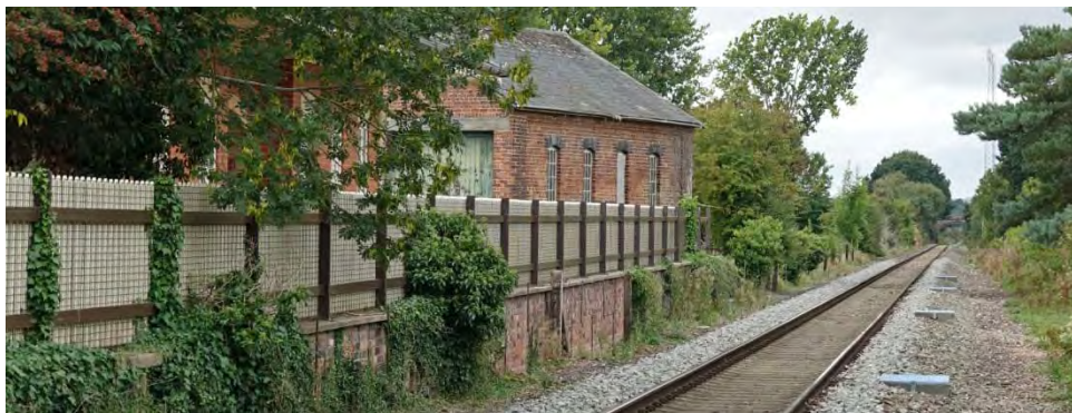
below looking west along the mainline towards Hereford from the level crossing (automatic half barriers) showing the re-built platform and goods shed, the line was singled in 1984 when the signal box which stood adjacent the station masters house by the level crossing was also demolished
