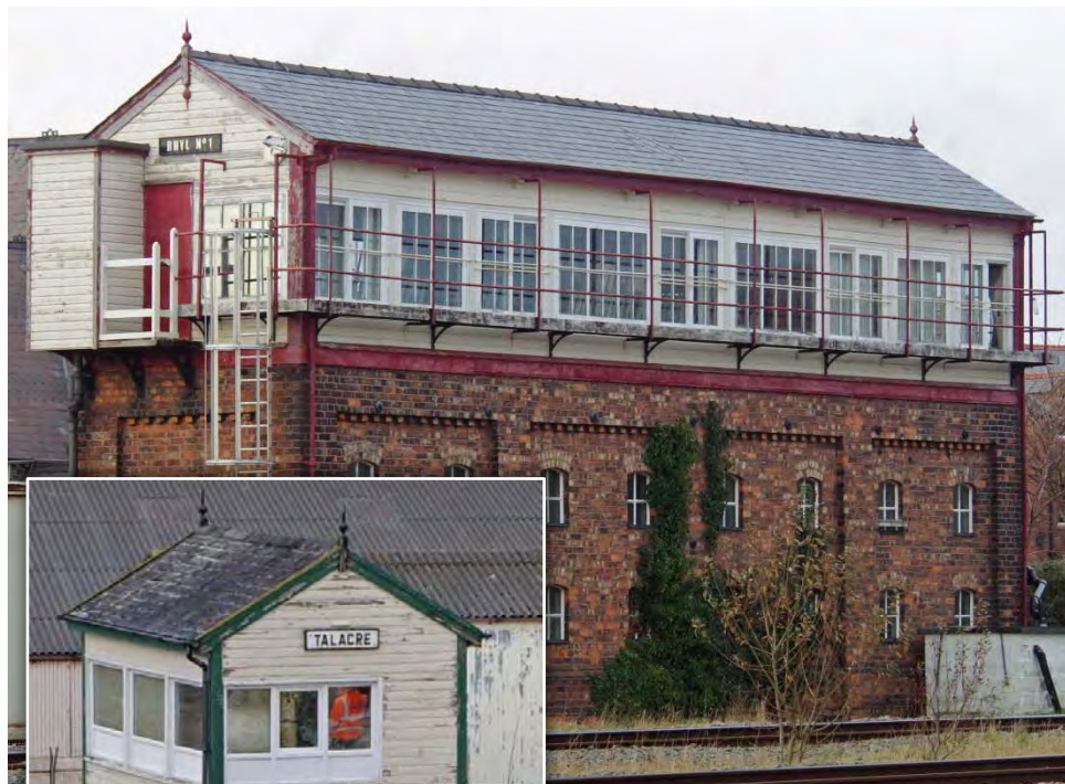
Mostyn: Situated between the tracks alongside the A548 on the access road to Mostyn Quay. Opened in 1902 it is a LNWR Type 4 box with a Saxby & Farmer 40 lever frame. It has an overhanging design (photo below taken by Darren Pavitt, 27 th January 2018).
