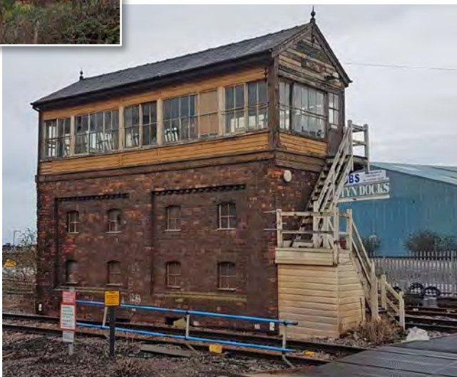
Mostyn: Situated between the tracks alongside the A548 on the access road to Mostyn Quay. Opened in 1902 it is a LNWR Type 4 box with a Saxby & Farmer 40 lever frame. It has an overhanging design (photo below taken by Darren Pavitt, 27 th January 2018).
