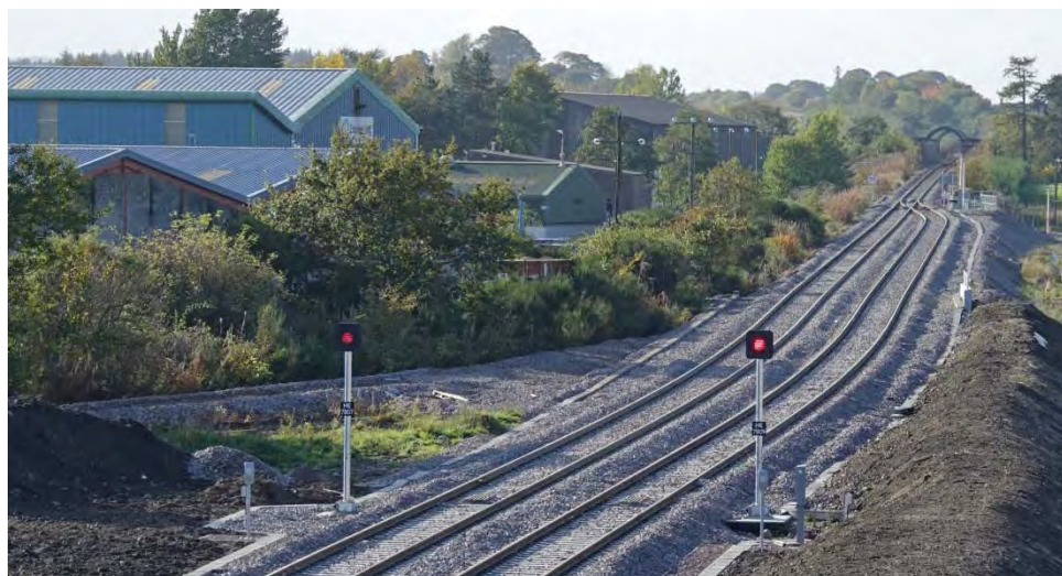
above looking west from Benromach Way showing the change from double track to the previous single track to cross the River Findhorn and the previous single track alignment on the left, 21 st October 2017
