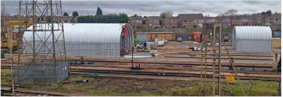
above seen during construction, 12 th January (Simon Sims)
