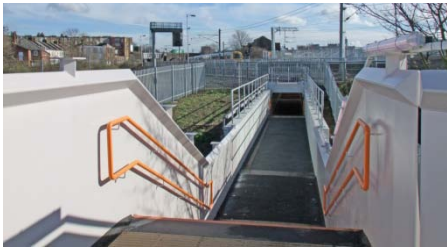
the walkway from the LL overbridge above platform 3 looking east towards subway under HL platform 4, 14 February 2011
