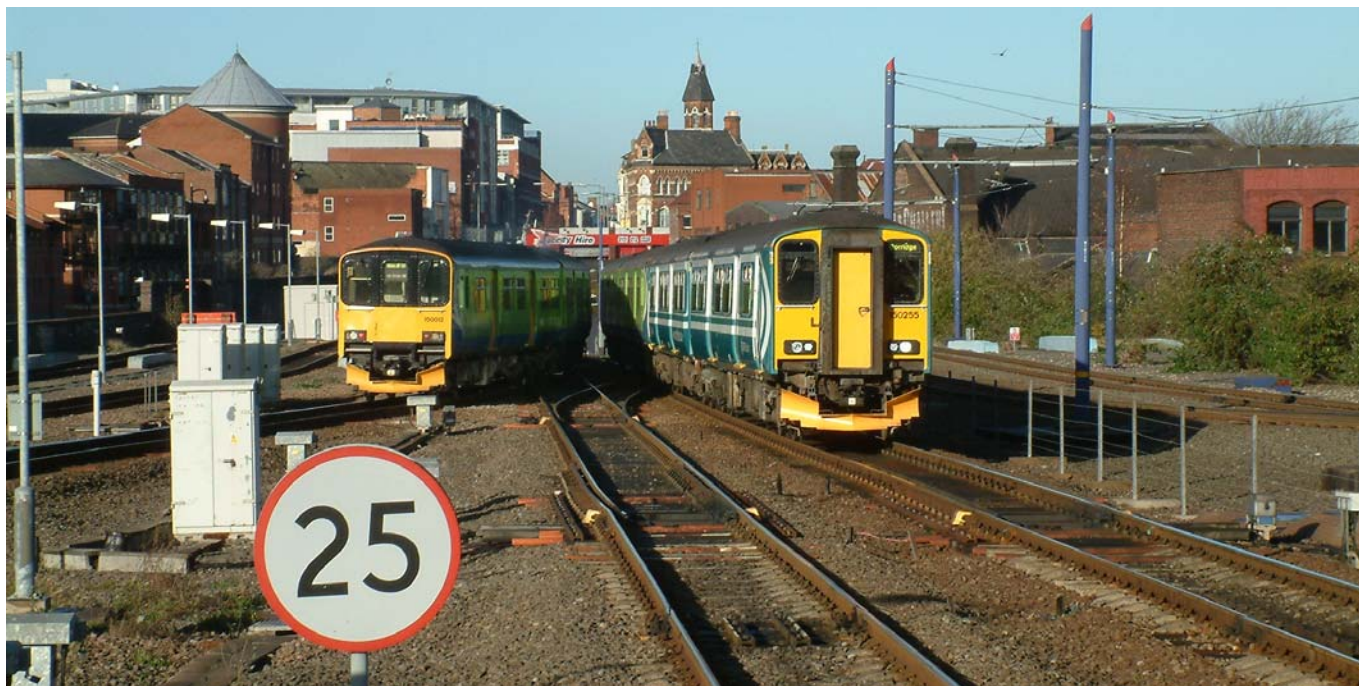
Centro 150112 & 150255 departing platform 1 and approaching platform 3 respectively looking north-west from end of platform 1 / 2, Metro tram track on right B'ham Snow Hill, 28 November 2006
